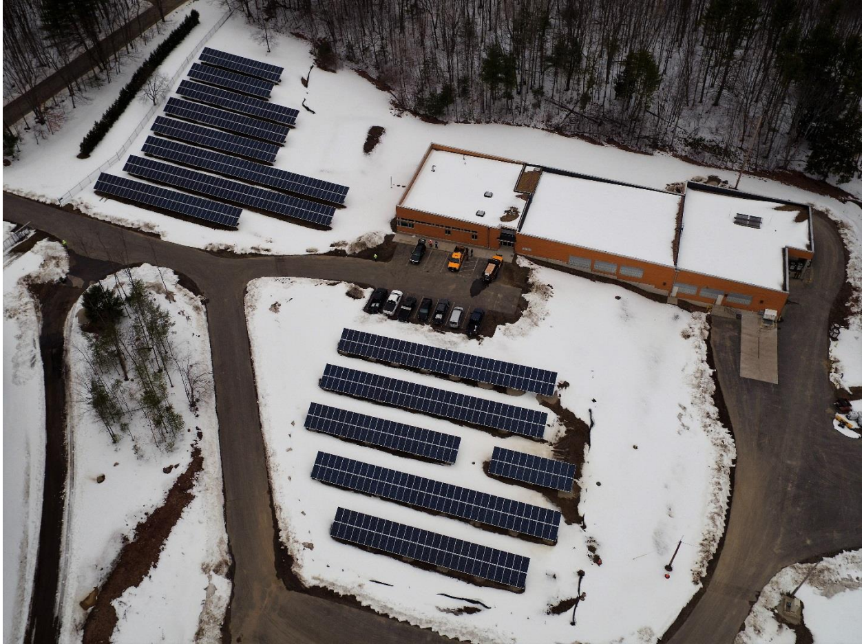
Madbury Water Treatment Plant
