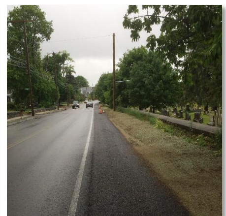
Sagamore Ave. Reconstruction with Porous Pavement
