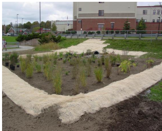
Rain garden, Portsmouth High School
