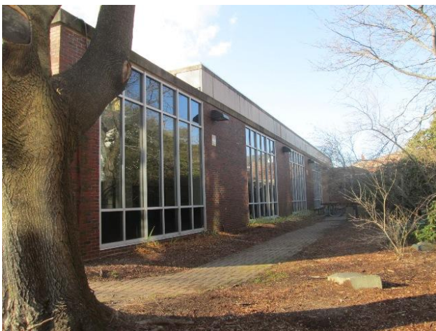
Photo 6 East elevation of one-story wing
