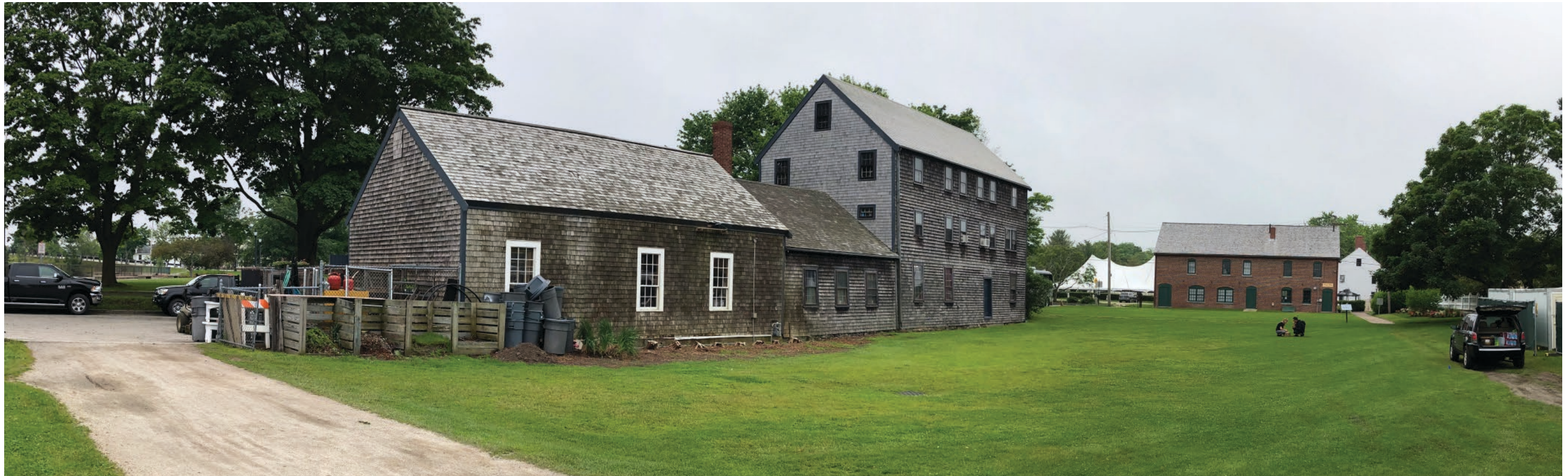
View of existing buildings: Garage/Lean-to/Shaw
