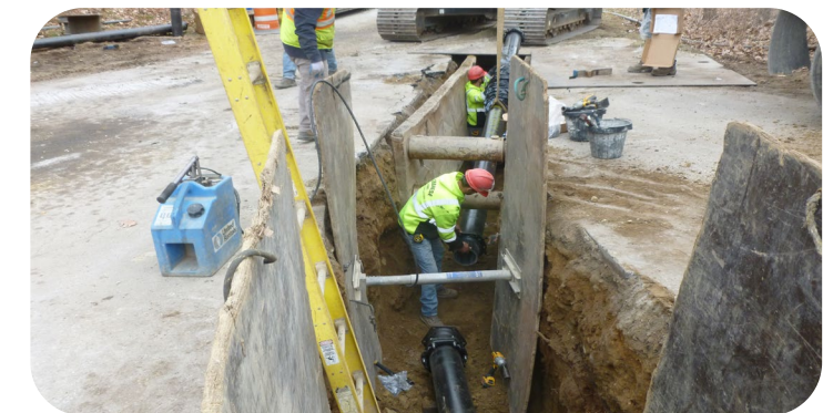
Tie-in connection on Lavenger Rd. (2022)
